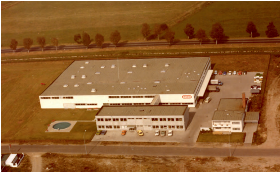
The new plant site in the Hanau industrial area in Germany shortly after completion
