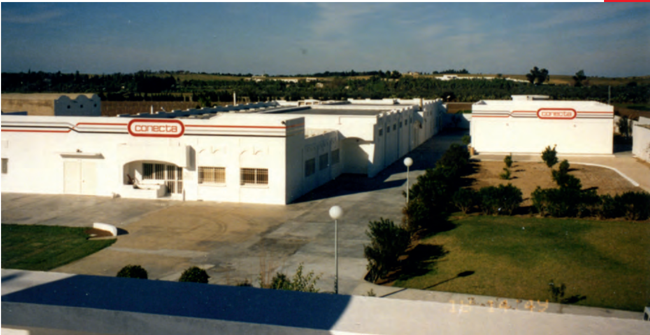
The company site in Tunisia 1981
